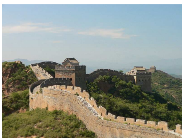
Pass the rice mortar: The Great Wall of China is held together by sticky rice mortar – and even today it remains the best available material for restoring ancient masonry.
